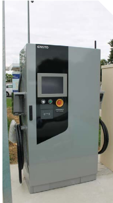
Station de recharge rapide
